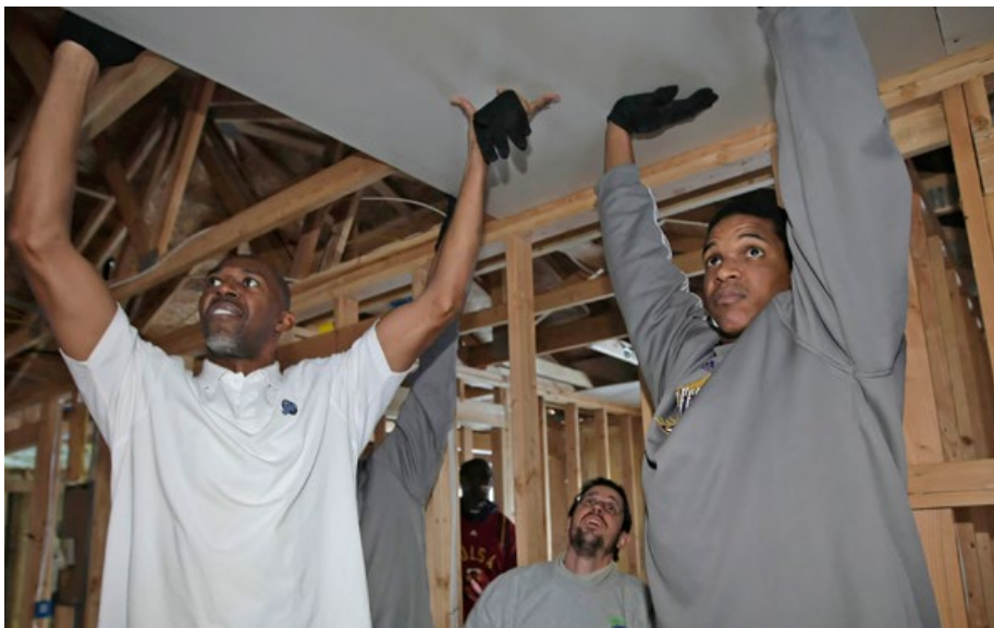
G-League players with the NBA, WNBA, Utah Flash and in partnership Habitat for Humanity, work on building a home in Provo, Utah on January 7, 2009. Habitat for Humanity is building a disabled accessible home for Galen and Victoria Sorensen and their two young children.
